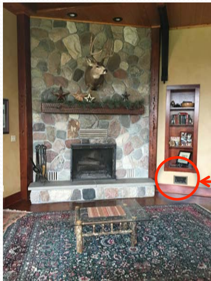
Supply Vents Added at 2 locations
